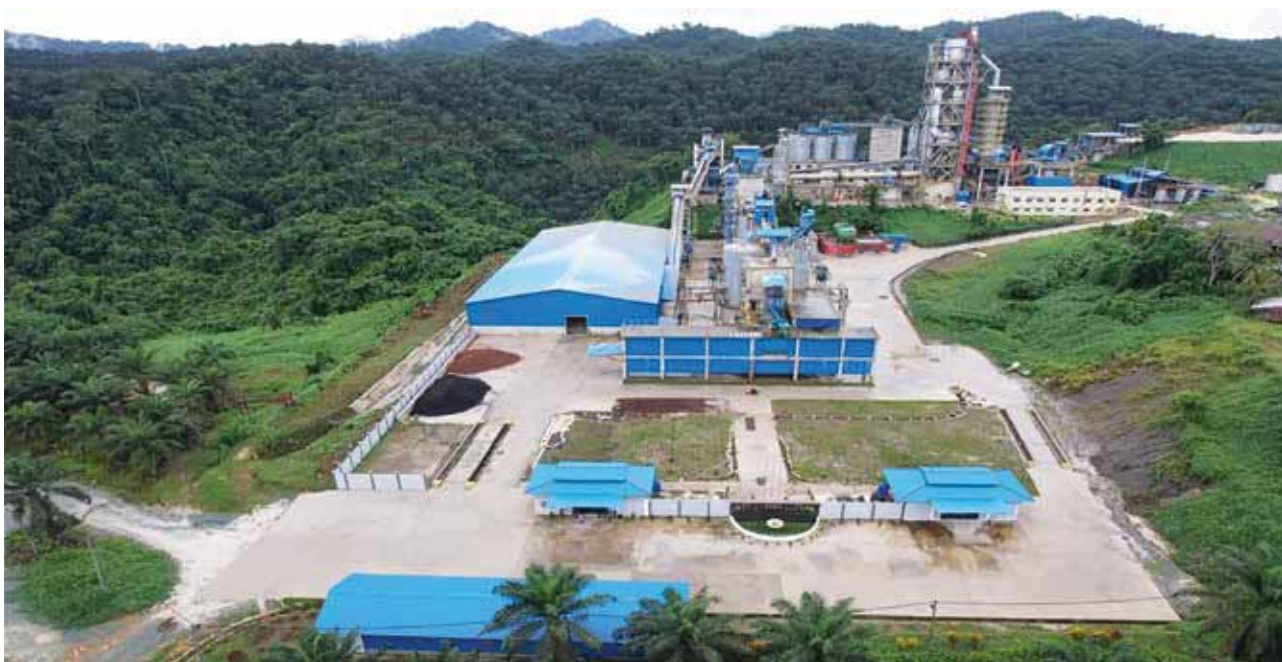
Aerial view of Integrated Limestone Processing Plant
