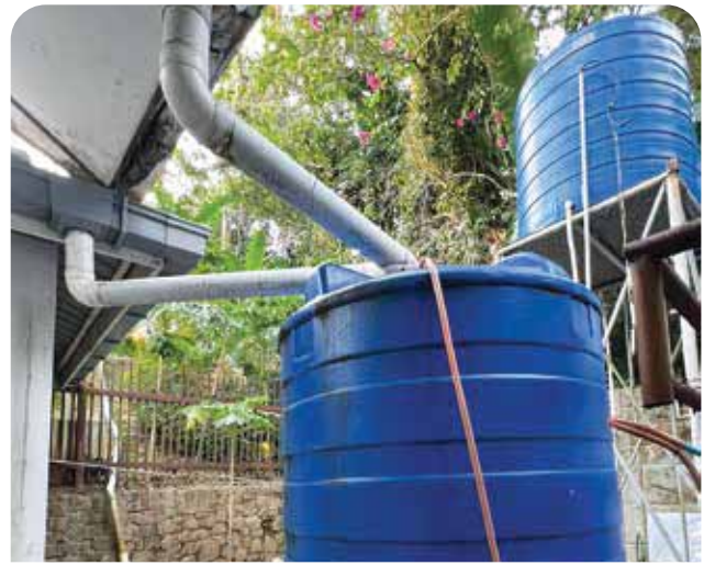
Rainwater collection system at one of the Staff Quarters supporting the Group's sustainability goals.
