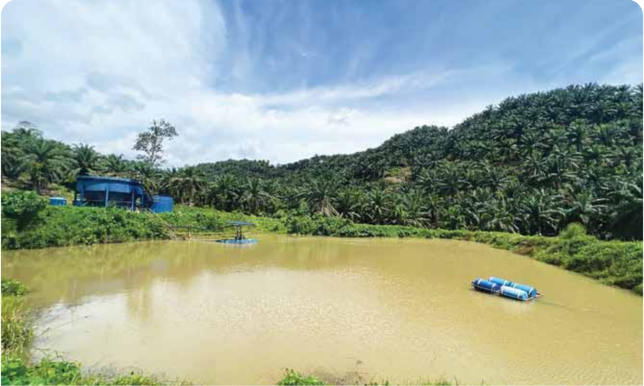
Rainwater harvesting system implemented at one of BOB's facilities, utilising rainwater sources for various operational needs.
