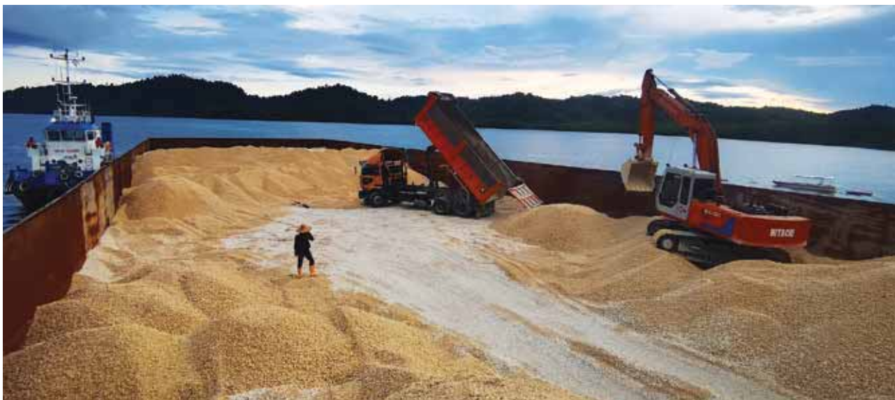
Limestone aggregates loading
